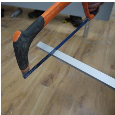
Cut the H Section to the required length and place it back upon the lower partition panel.
