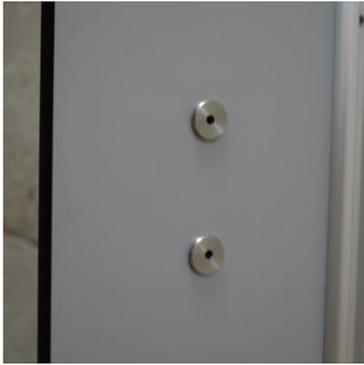
Fit the smallest piece of the separated hinge to the pilaster. So that the pins point up, this allows you to fit the hinged channel and door by dropping the assembly onto the hinges.
