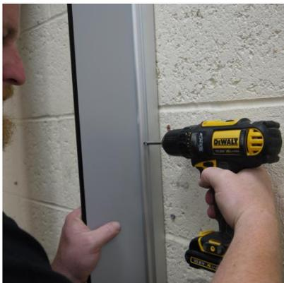
Drill pilot holes for the screws.
