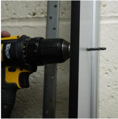
Starting with the second smallest drill bit (4.5mm) drill all the way through the panel at the correct place.
