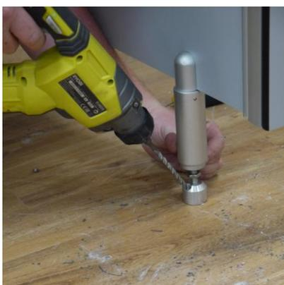
Pull up the collar on the cubicle legs exposing the drill holes.
