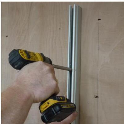
Fit the channel drilling pilot holes for rawl plugs if required.
