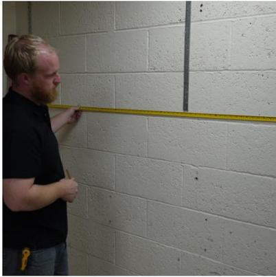
Measure out the position for the wall channels on any side walls. These wall channels will attach the wall pilasters to the side walls.
