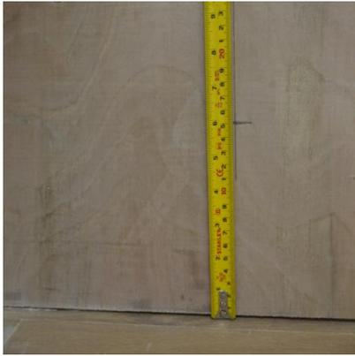
Measure up 150mm from the floor and add another mark. This is the height at which the panels are raised from the floor and from where the channels should be installed.
