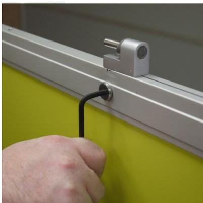
Returning to the pilaster we now need to drill the holes for the bolt through fixings which will attach the hinges.
