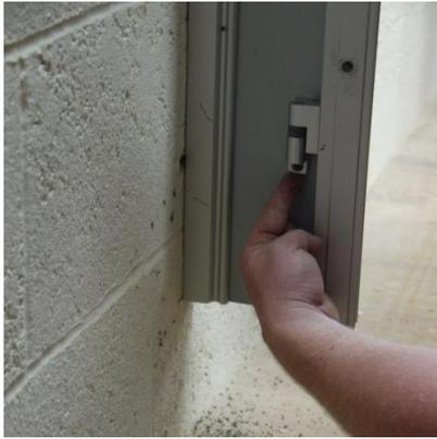
Offer up the hinge to the pilaster. Ensure it is on the inside of the cubicle and on the side the cubicle will hinge from.
