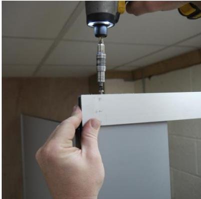
**Pilot holes must be drilled for ALL fixings fitted in or through compact laminate material!**
