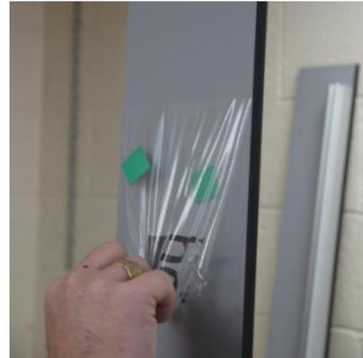
We will start by fitting the last pilaster this is our terminating pilaster and is on the corner of the cubicle set.
