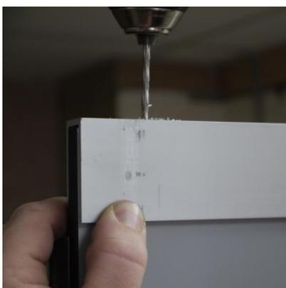
Starting at the corner end drill pilot holes for the screws.
