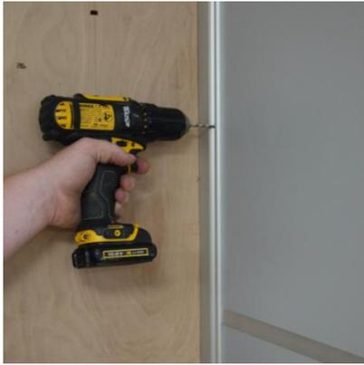
At the wall end drill pilot holes for the screws.
