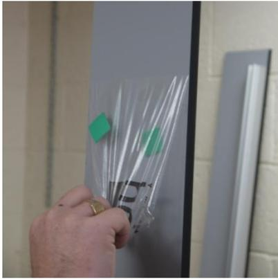
Preparing the wall pilaster for use we once again clear it of protective material.
