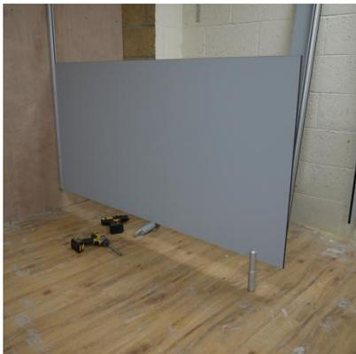
As before pilot drill each hole before using the supplied zinc screws to secure the panel within the wall channel.
