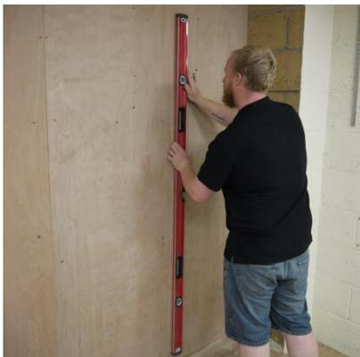
Measure out the position for the wall channels using the information supplied in your drawings.
